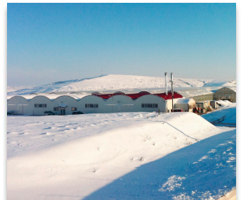
RUMANÍA Invernadero APG96r APG96r Greenhouses 3 Has.
